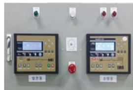
Fire Feeder Digital Type(GCP i7 + fFD)
